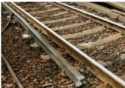
Conductor rails (third rails) provide trains with up to 750 volts DC. The live rail is raised on insulating pots. Cables attached to these rails must be considered to be live as well.
